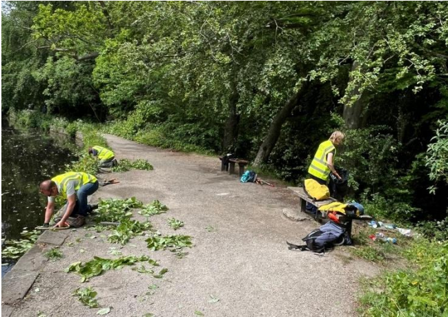
Cutting back at Havelock Dam
