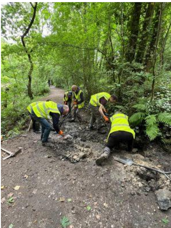
Volunteers backfilling the trench at Holme Head and diverting a stream into an existing drain.
