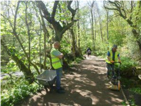
Compacting the footpath material at Holme Head. Photo: Scott Berg
