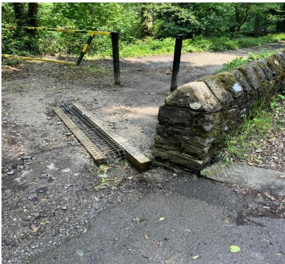
The completed floodwater diversion at the top of Nether Cut drive at the S bend.
