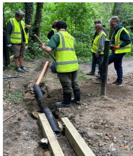
Installation of the flood water diversion at the top of Nether Cut drive.
