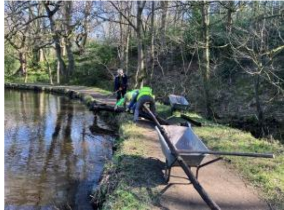
Removing logs and debris from Hind Wheel dam. Photo: Roger Kite
