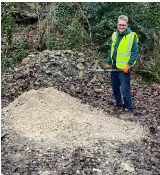
Andrew eking out the remaining footpath material left at Hind Wheel.
