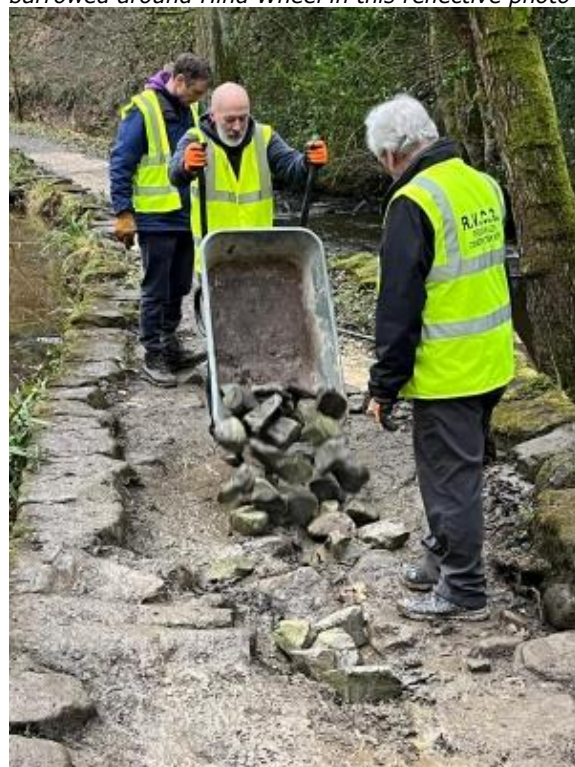
Large stones are used to fill the footpath voids before being covered in finer material.
