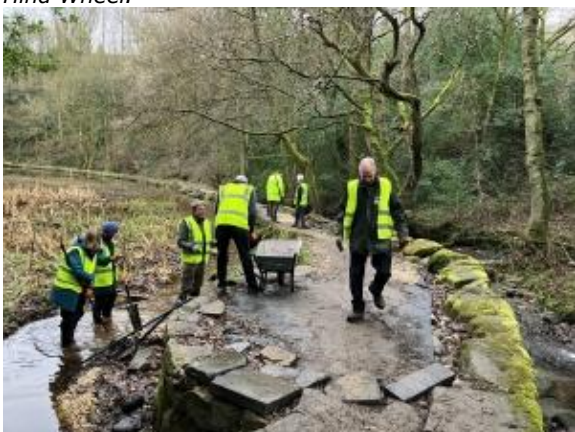
Hind Wheel: Volunteers recover footpath material swept off the footpath and into the dam in a recent storm. Photo: Roger Kite
