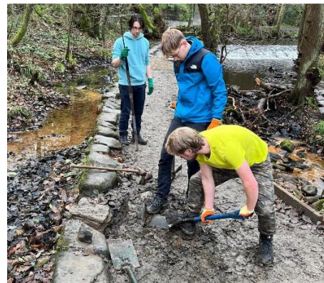
The footpath is prepared for its topping of sandstone
