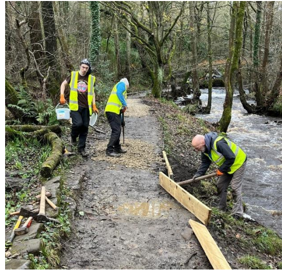
Kevin and Ed install revetment boards to contain the sandstone.
