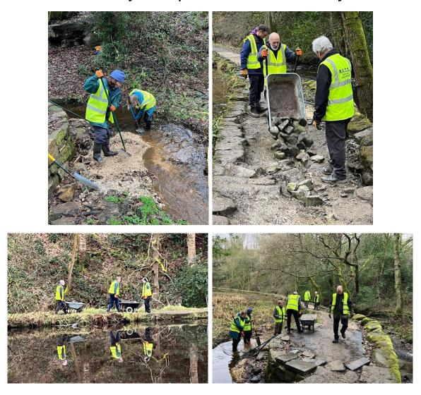
The RVCG Task team was out in force on Sunday 26<sup>th</sup> January 2025 working to make repairs around Hind Wheel. This involved barrowing a huge amount of stone and path topping material to level and repair the footpath around the dam damaged in recent storms. The goit at Hind Wheel had also become clogged and so was cleared. Thanks to all who took part helping that day.
