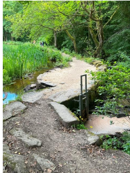
June 24 Hind Wheel (West) repaired by Sheffield City Council
