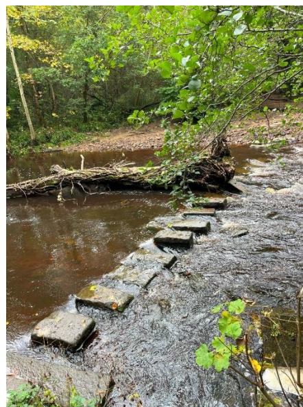
The recently restored stepping stones at Roscoe Wier have been dislodged by this tree washed down during the flash flood.
