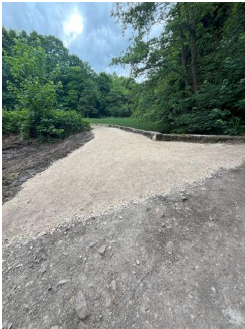
June 24 Hind Wheel (East) repaired by Sheffield City Council
