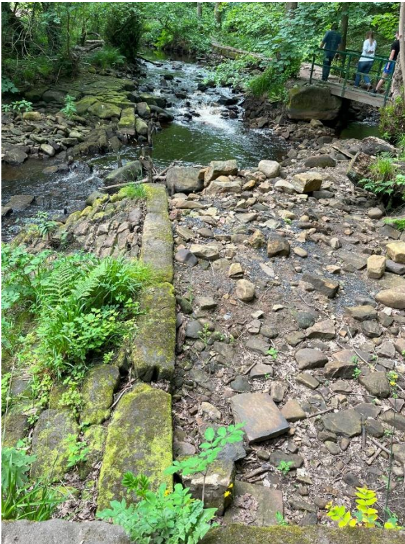
Swallow Wheel head goit completely blocked with grit and rocks and showing the weir washed away in the background. There is no water flow here anymore and sadly the dam will slowly dry out.
