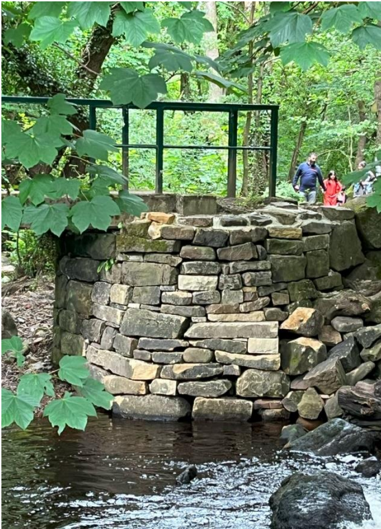
Sheffield City Council repairs to the foundation of the bridge at Hind Wheel
