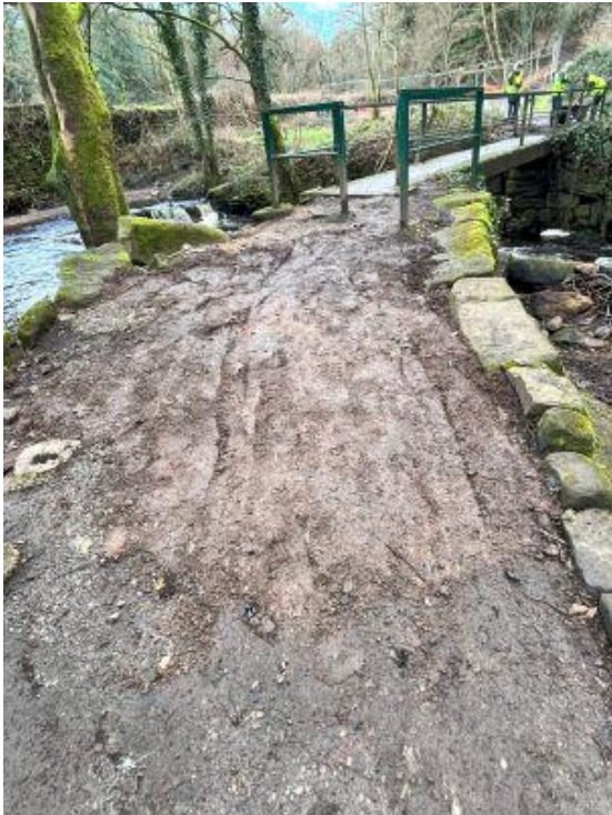
Pathway resurfaced at Hind Wheel bridge
