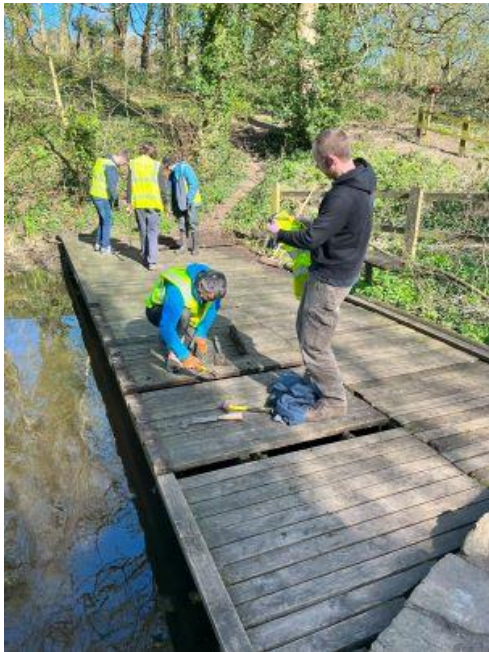
Task team volunteers replacing rotting timbers at Rivelin Corn Mill dipping platform
