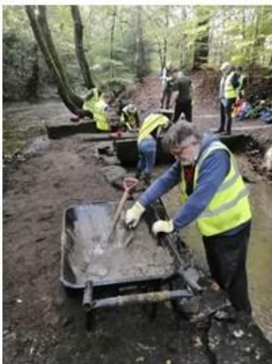
Frank goit wall restoration (Hannah Isherwood)
