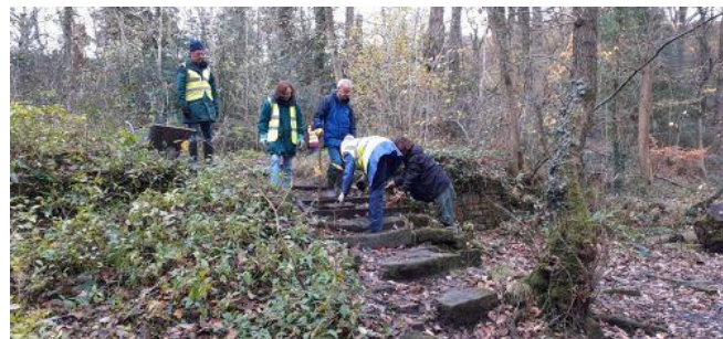
Restoration of the steps at 2 nd Coppice (Sue Shaw)
