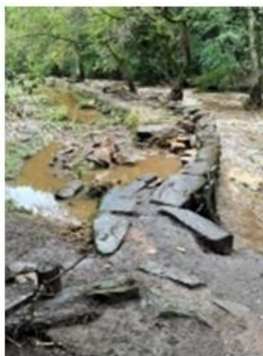
Serious footpath damage at Hind Wheel (West)
