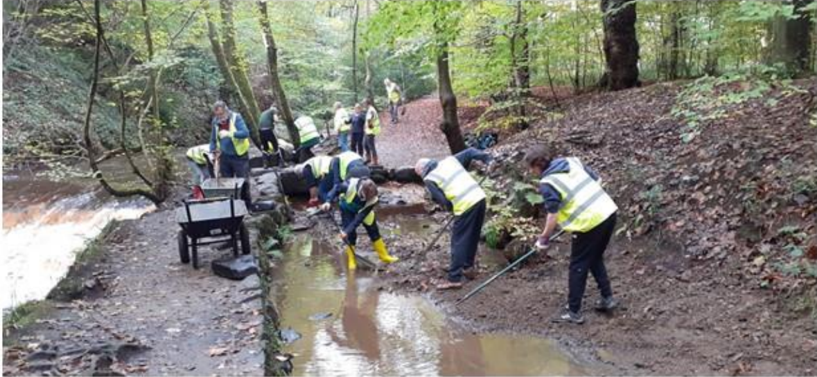
Silt removal at Frank goit (Sue Shaw)
