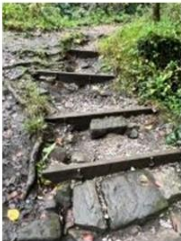
Second Coppice Steps washed away
