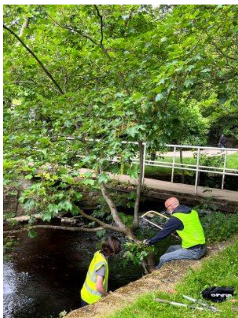
Trimming back the trees growing in the riverbank
