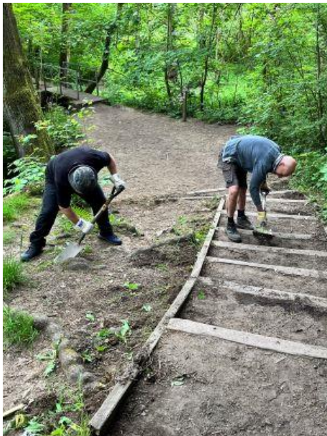
Restoring the steps at New Dam
