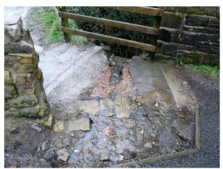
The same entrance after task day. Wall repaired, drain installed, footpath repaired
