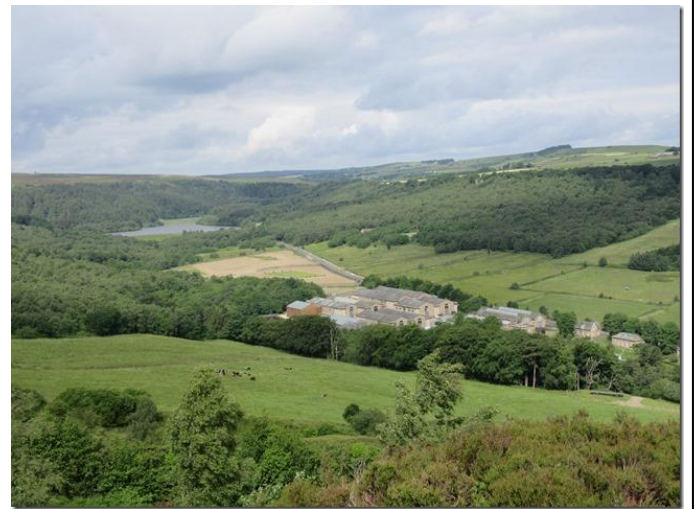
Figure 2. In this wider view the new building is completely invisible thus achieving our desire to minimise the disruption to the scenic view.
