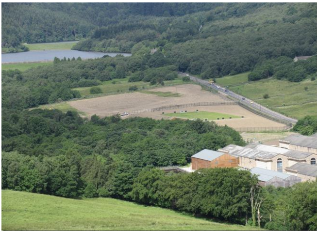
Figure 1 At RWTW the new two-storey building is almost invisible; just picked out by the green square in this picture
