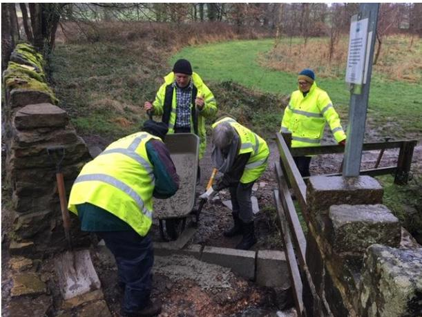
*A new sill is concreted into place and a new waterway created for flood water.*
