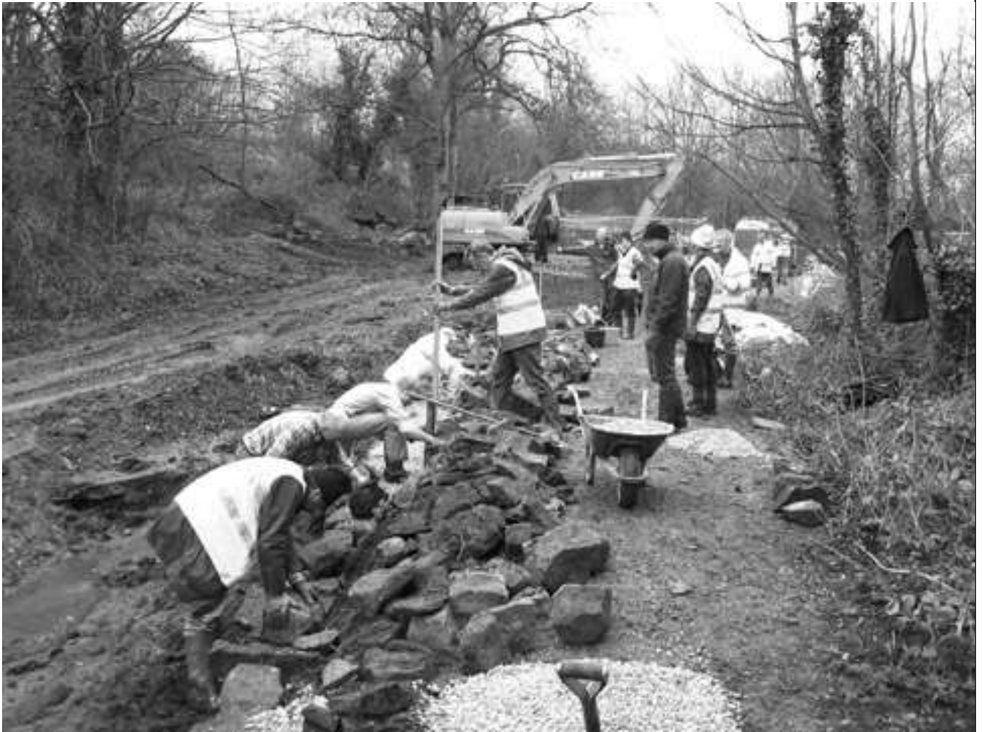
The RVCG task team at Rivelin Mill Dam.
